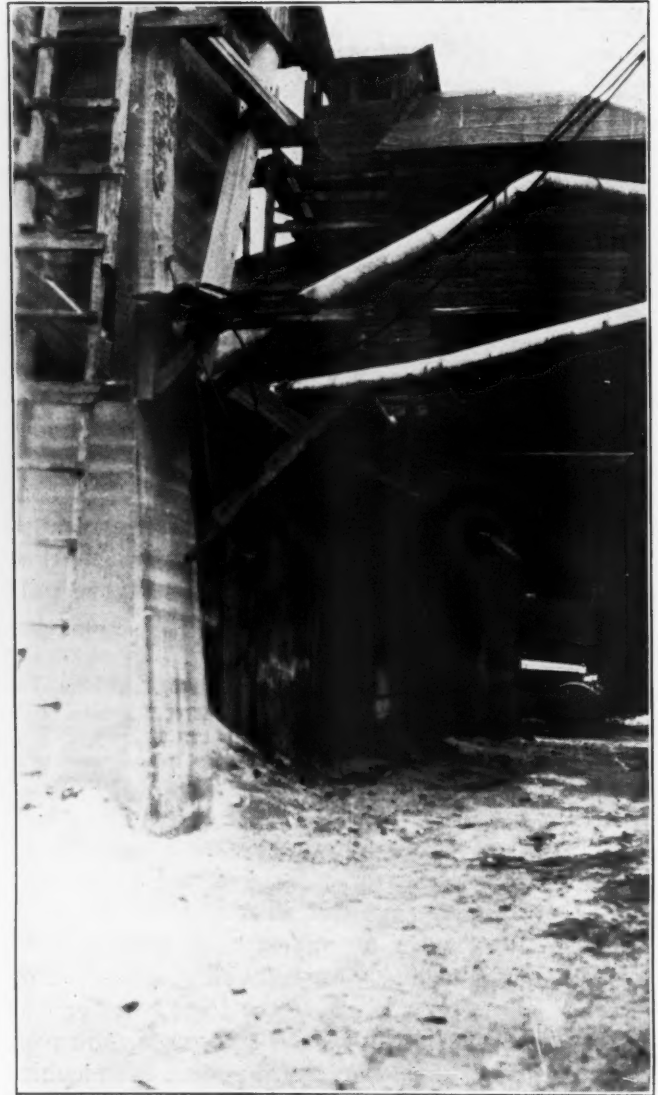
Crushing Plant at Left and Storage Bins. Pipes are Part of the Dust Collecting System.
